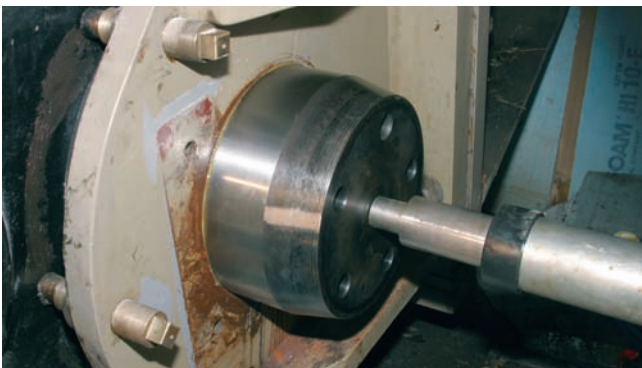
The hydraulic jack slides the shaft into position.
